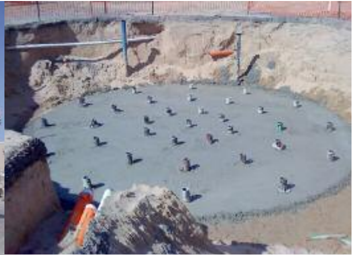
Navigation Tower Footings
